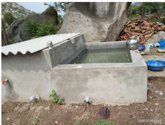
Figure 13 Tank for irrigation
