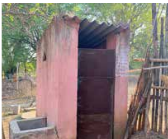
Household Toilet, Mayurbhanj
