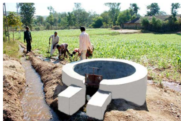
Lift Irrigation Outlet point of Boriya Lift Irrigation Cooperative, Panchmahal, Gujarat
